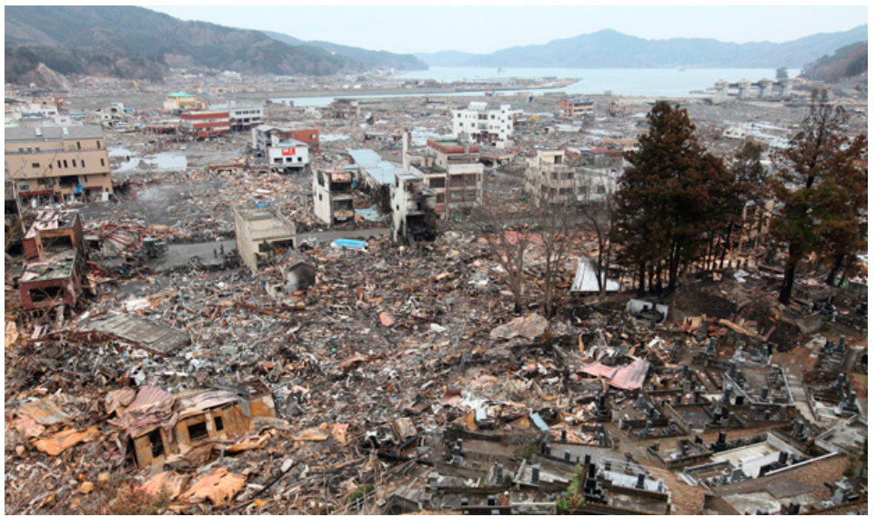
Figure 6: aftermath of tsunami impact.
